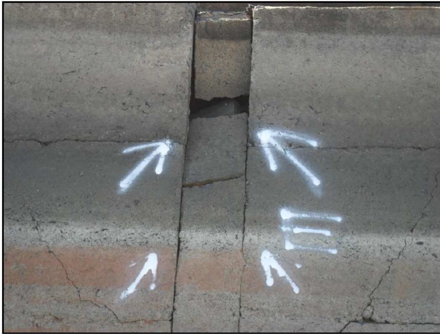
Figure 6 - Honeycombing of Concrete on Existing Rehabilitation Work
