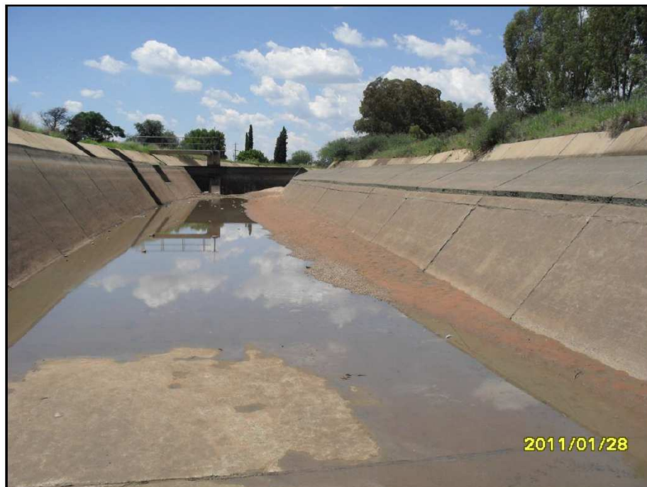
Figure 4 - Sedimentation of Eroded Soil in Canals
