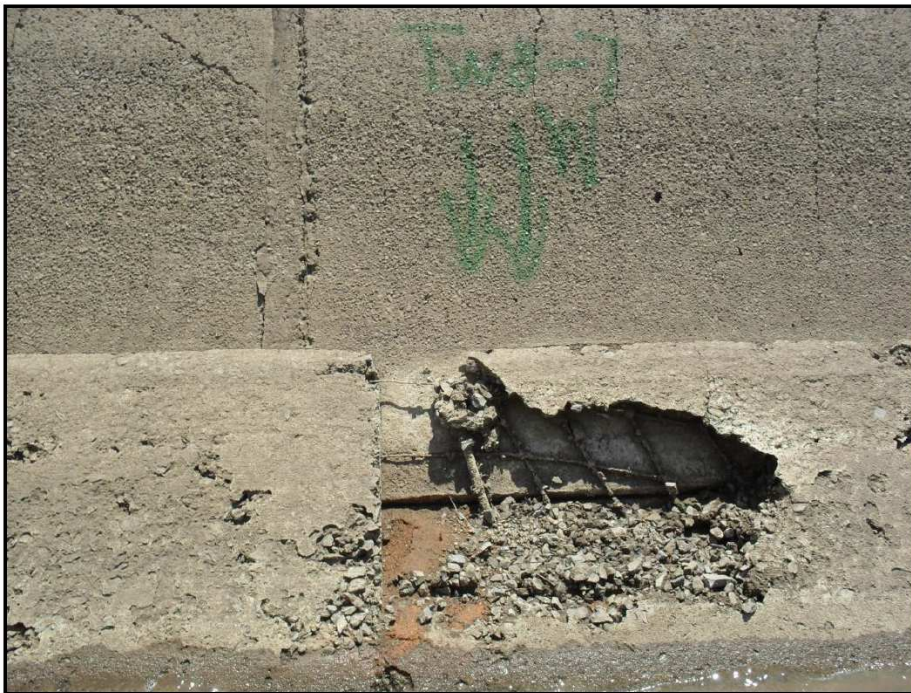
Figure 6 - Honeycombing of Concrete on Existing Rehabilitation Work
