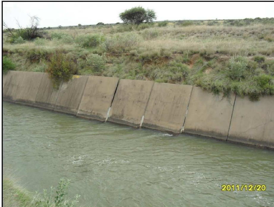
Figure 3 - Cracked Canal Lining
