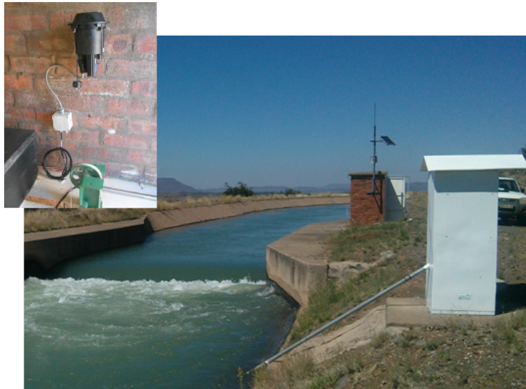
Figure 2.1: Scheiding measuring station with Cello logger
