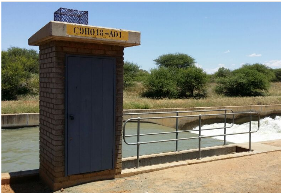
Figure 10.5: Measuring station at Vaalharts main canal
